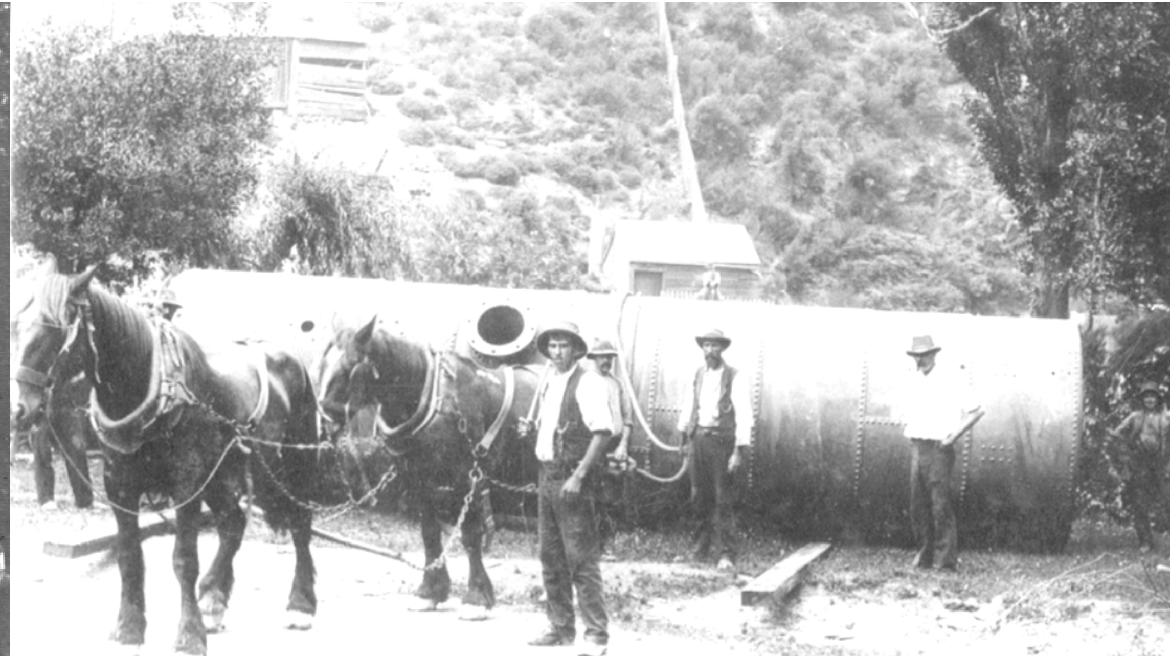
Photo: Horse team on the road from Jamieson hauling a boiler for the use on the goldfields. From Tomlin O.F., Bosa M., Chamberlain P.G., 1979, 'Gold for the Finding: A pictorial History of Gippsland's Jordan Goldfield'
