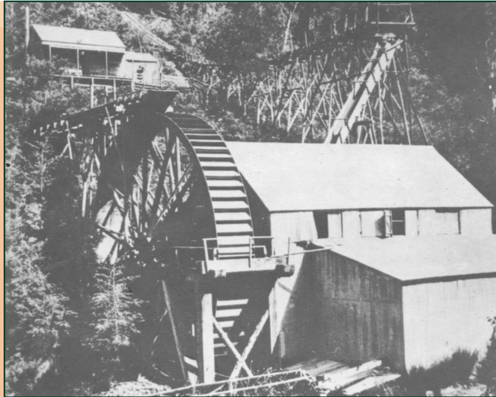
"A water wheel situated near Woods Point, similar to the construction that would have been used for the Golden Wall crushing machine c.1905"
