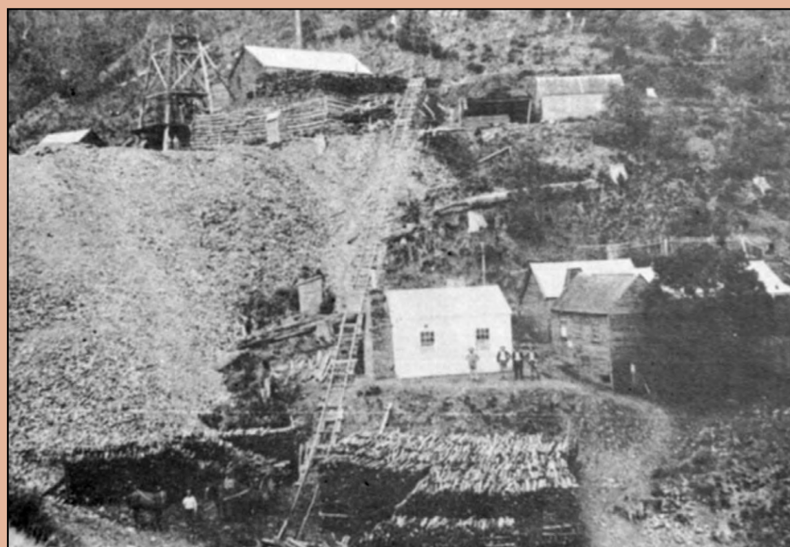
Toombon mine, showing shaft, mine managers house and surrounding mine buildings, note large supply of firewood to fuel the boiler c. late 1800
