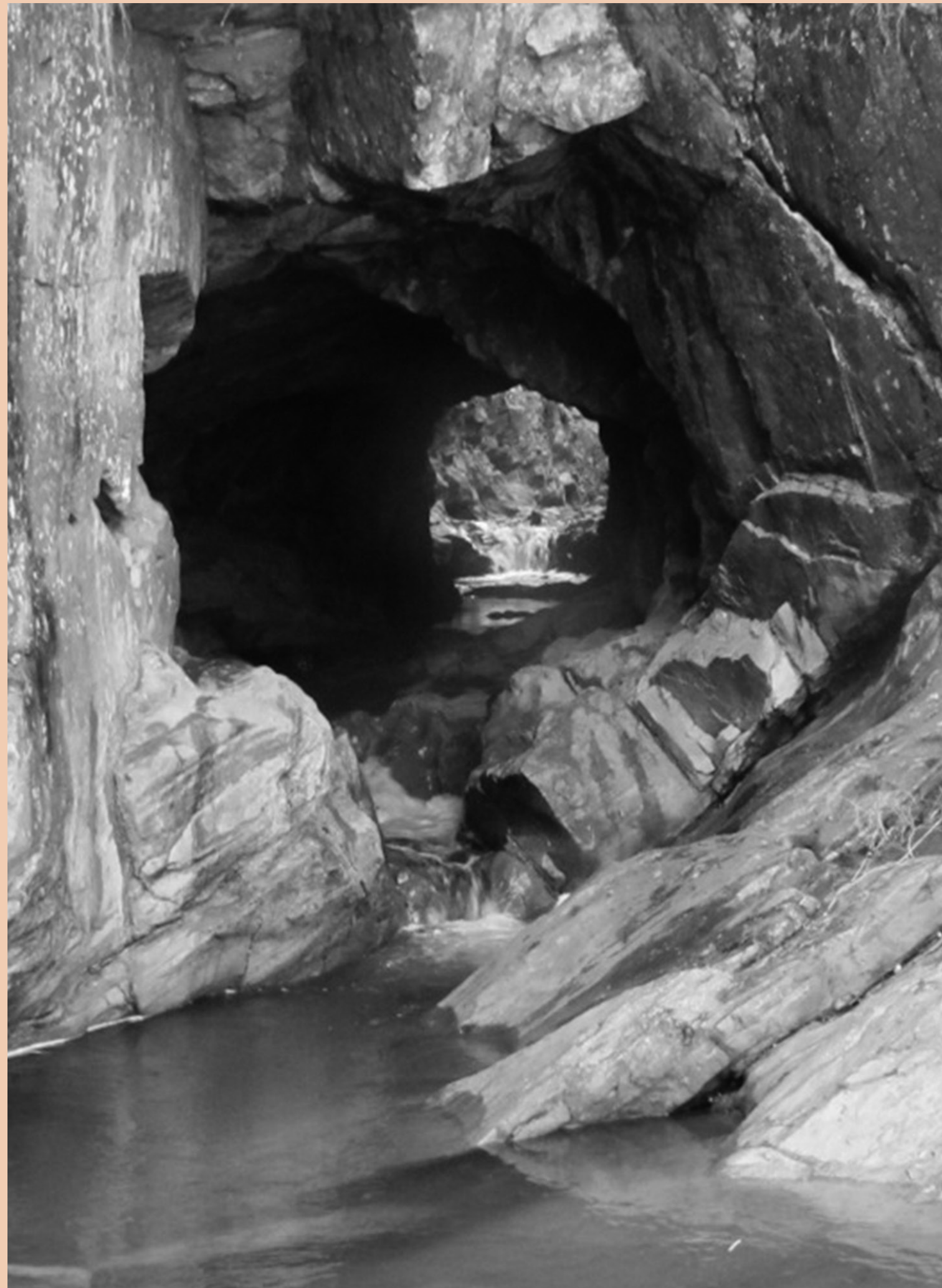
Entrance to the diversion tunnel as it is today.
